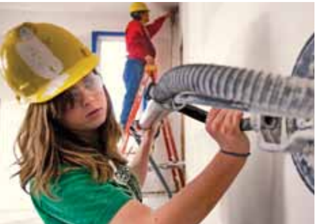
A high school student learns sustainable trade skills as her team helps rehabilitate a home in Dubuque's Washington Street neighborhood. (Four Mounds Foundation photo)
